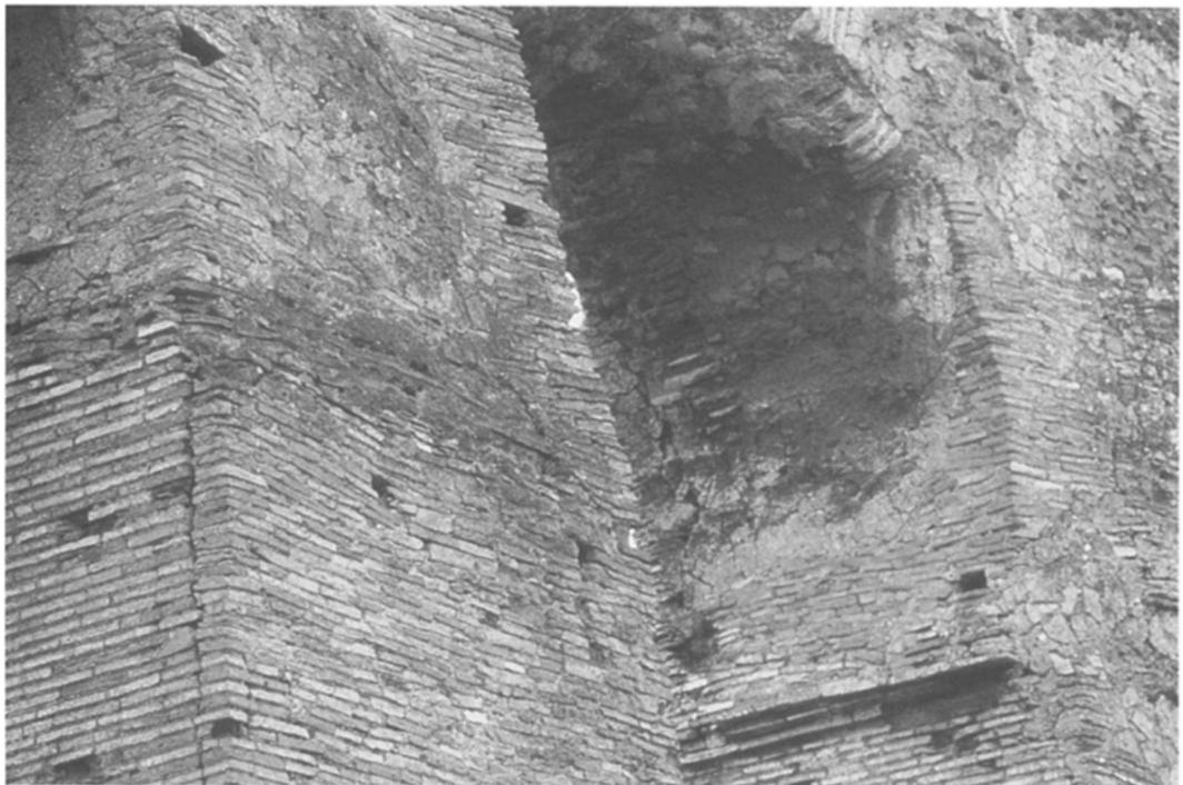
2. AQUA ALEXANDRINA AT TOR TRE TESTE. ARCADE REBUILT IN RE-USED BRICK.
