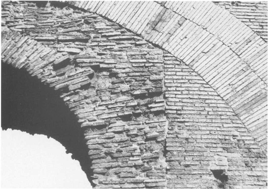
1. AQUA CLAUDIA IN THE VILLA WOLKONSKY. SUSTAINING ARCH IN RE-USED BRICK.
