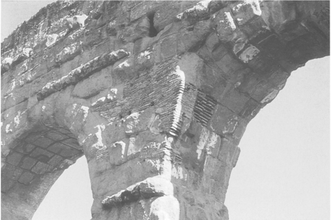
1. AQUA CLAUDIA AT CAPANNELLE. PATCHING IN RE-USED BRICK.
